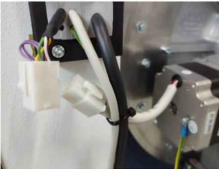
Disconnect the loader wheel motor plug. If there is no plug, the cable in the control cabinet must be disconnected.
